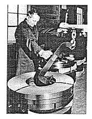
Placing spacer blocks between stacked coils permits easy insertion of the wedge. Lightweight and pivoting wedge makes it easy to position the hook.
