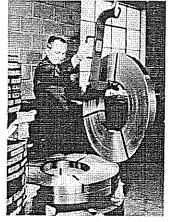
Coit is in vertical position after being lifted from its pallet. The weight of the coil holds the pivoting wedge in the vertical position during transportation.
